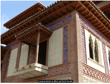
Architectural detail of West and South facade
